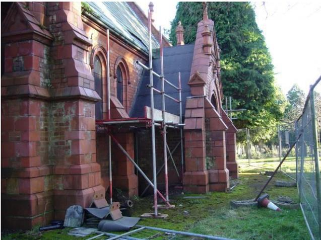
In January further maintenance work commenced on the Chapels and is ongoing. The roof of the Chapel with the least damage is being made weatherproof and the other, will have a temporary roof installed subject to planning permission. This is not a renovation project but an attempt to prevent further deterioration.
