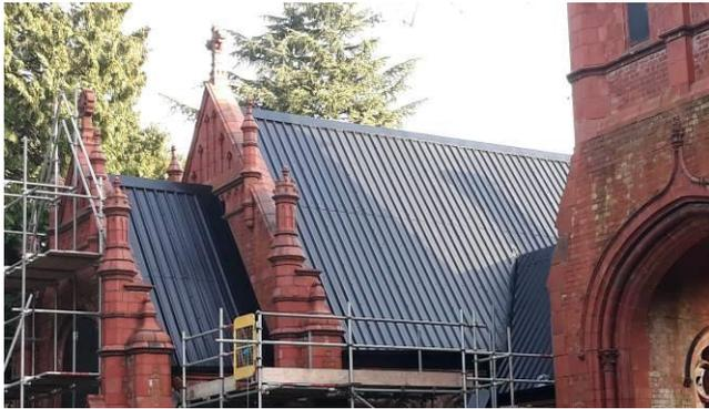
The installation of a temporary roof on one of the chapels is now complete. Although this is only a step towards preventing further deterioration, it is nevertheless a huge improvement to the appearance of the chapel.
